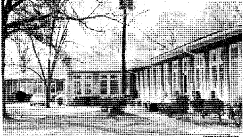
This is the rear of Bldg. 5 today. The portico in the 1926 picture was located where the two bushes in the center of the picture are.
