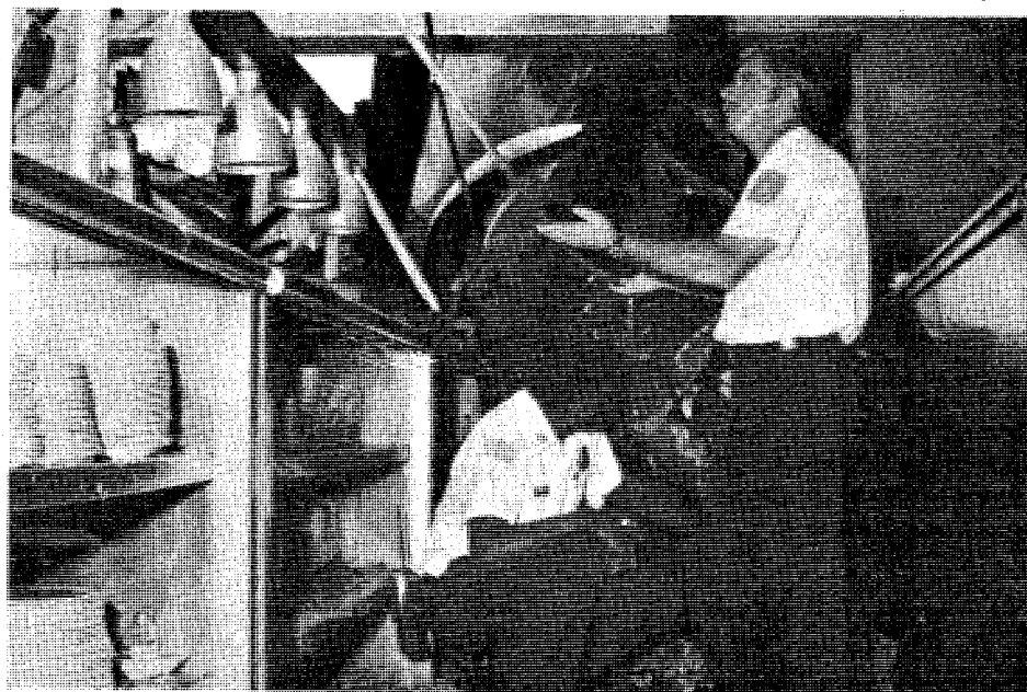
Benning fire inspectors James E. Floyd (standing) and E.J. Robinson examine fire damage.
